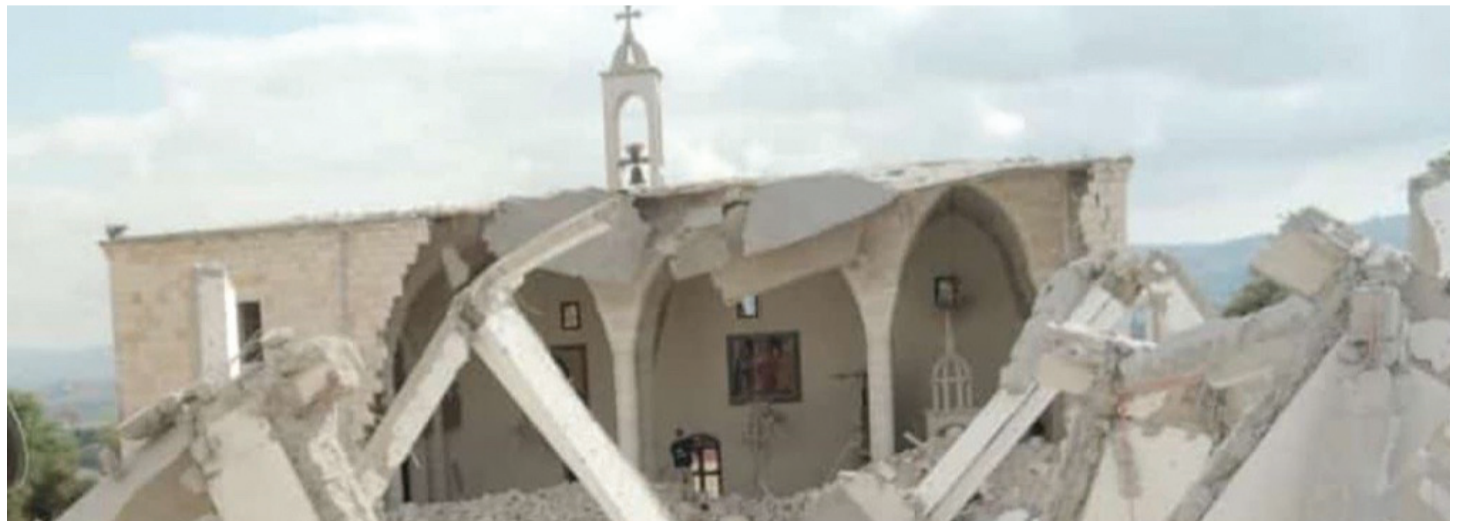
The destroyed church where at least eight people were killed in an airstrike – Photo © ACN
