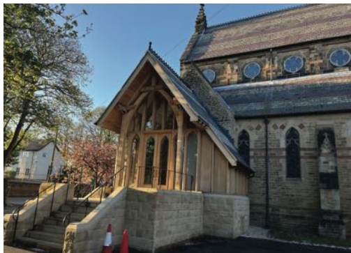
The new porch extension at St Wilfrid's Church, Ripon
